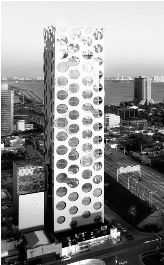
Figure 10: COR Building (Courtesy of Chad Oppenheim and dbox).
