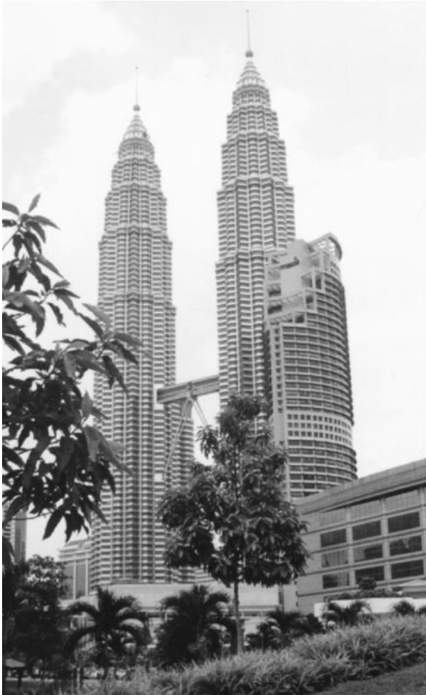
Figure 14: Petronas Tower (Courtesy of Abbas Aminmansour).
